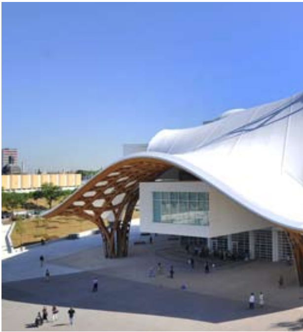
Figure 6. Centre Pompidou Metz with a roof surface as a wooden lattice adapting into a column.
